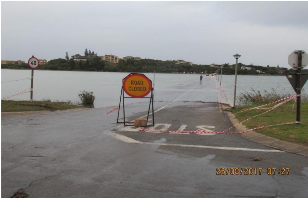
**Plate 8** Berm overwash shown in Plate 6 resulted in the causeway overtopping with seawater. Zero freshwater inflow to the estuary occurred around this time, so that salinity levels in the estuary would remain at 35 or higher. High rates of evaporation would rapidly result in hypersaline conditions developing in the estuary as the estuary closed again within 48 hrs. Photograph from Hennie Swanevelder – Department of Economic Development and Environmental Affairs.
